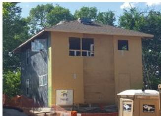
*Water/air/vapor control membrane applied.*
