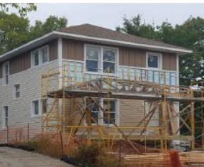
*Insulation, furring, and cladding installed.*
